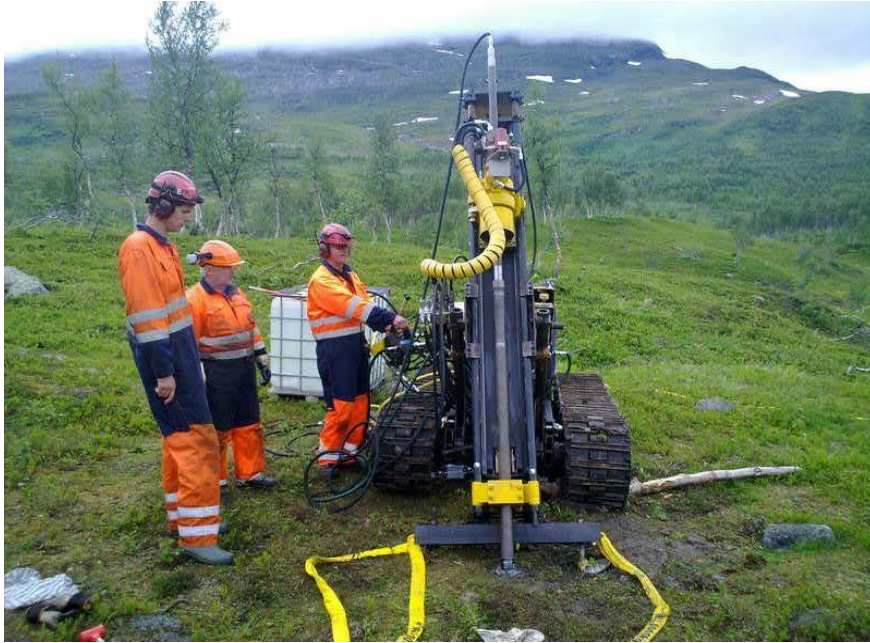
Figure 1 (a). Crawler Drilling Machine
