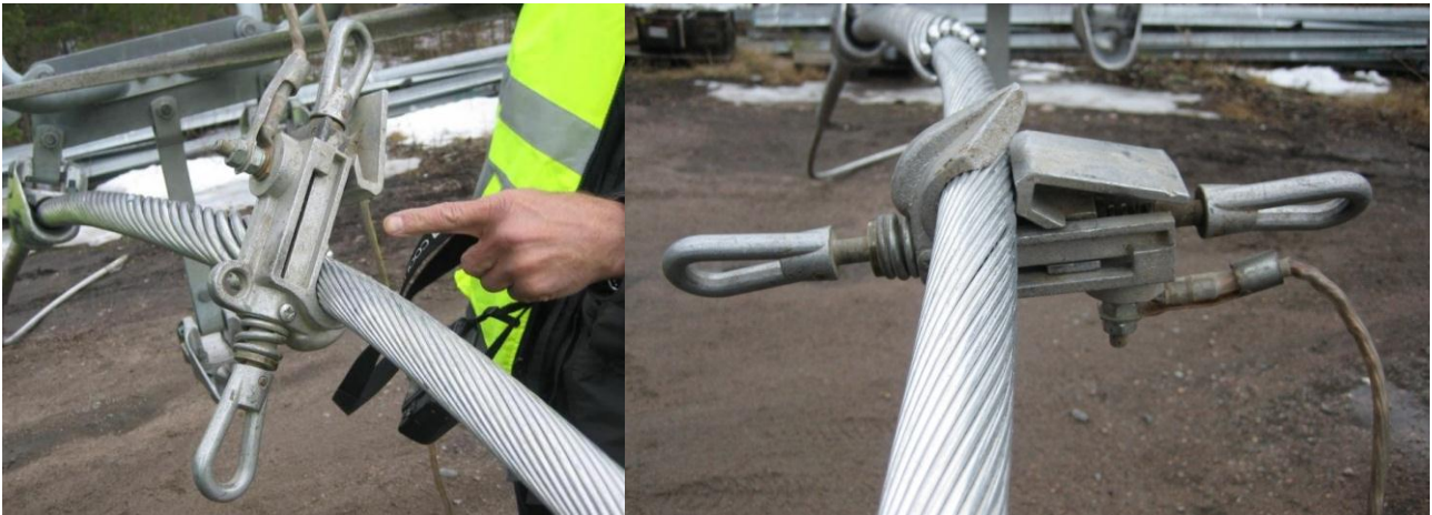
Figure 7. The picture on the left shows the line terminal tightened by pulling it onto the conductor, suspended by the earthing rope. The picture on the right presents the correct method.
